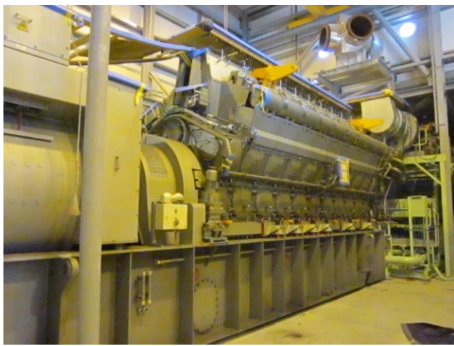
(ABOVE) An 18-cylinder engine attached to an 8.7MW generator during plant construction near Freeport, Bahamas (RIGHT-TOP) A new, natural gas-fired boiler in Halifax (RIGHT -BOTTOM) Refrigeration plant in Halifax
