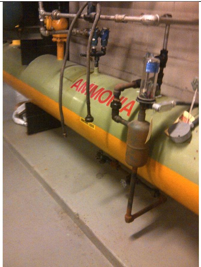
Above left: header carrying cold brine and tubes carrying brine beneath ice surface and tubes returning brine to return header. Above right: Ammonia receiver – yellow represents liquid and green represents gas.
