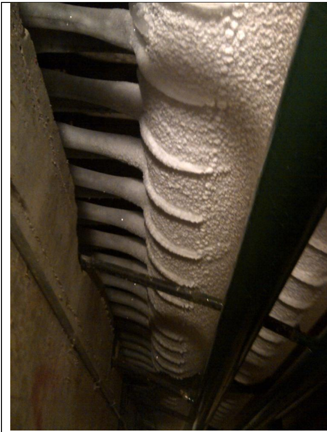
Above left: header carrying cold brine and tubes carrying brine beneath ice surface and tubes returning brine to return header. Above right: Ammonia receiver – yellow represents liquid and green represents gas.
