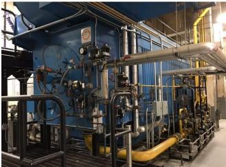
The VG Boiler Plant is a high pressure steam plant rated at 88,146 kw. The plant operates three 100 KPPH packaged water tube boilers at 120 psig drum pressure and 110 psig header pressure. Plant steam load will fluctuate between 20 KPPH during nights in the summer to 100 KPPH on the coldest days of winter.
